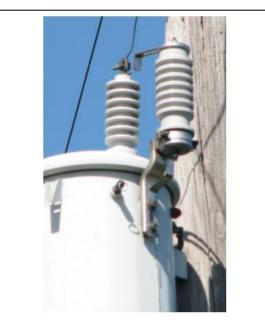
Figure 3: Surge current path through steel ground strap and steel tank
